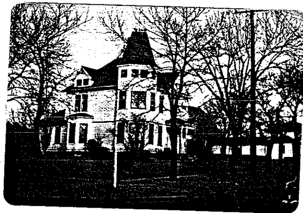
View From The Southwest
